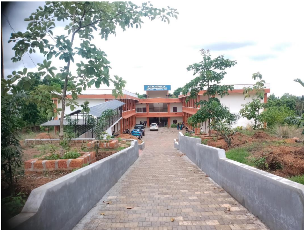
FIGURE 2: CAMPUS BUILDINGS VIEW
